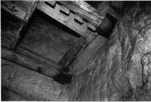
One of the ventilation shafts. Photo Tony Page
